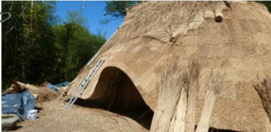
Rebuilding replica 1000 AD houses using traditional methods - wooden frame and thatch
