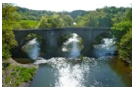
Kirkfieldbank three arch bridge
