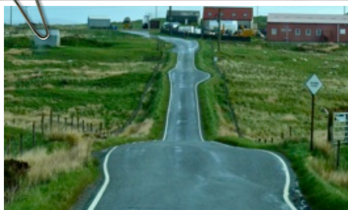
A typical one lane highway with passing lanes
