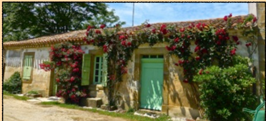
LOCK KEEPER'S RESIDENCE
