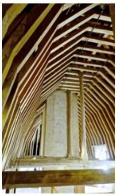
VAULTED WOODEN CEILING
