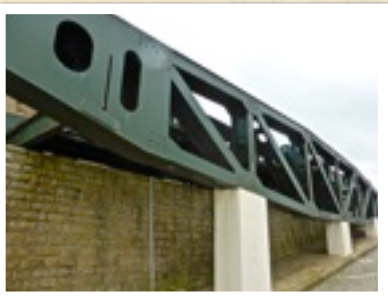
STEEL GIRDER BRIDGE
