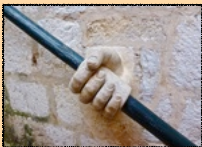
HELPING HAND As we were climbing up the stairs in one of the buildings we came across a guide rail fastened to the wall by this unusual sculptured holder.
