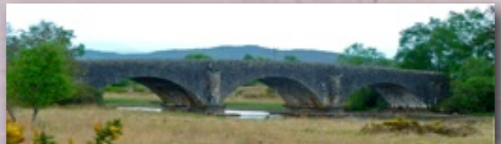
Old stone bridge on the road from Ardnamurchan
